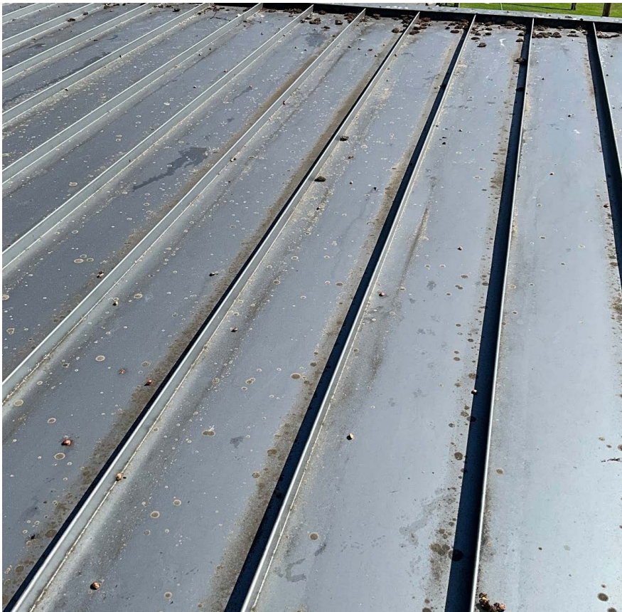
Condition of the roof
