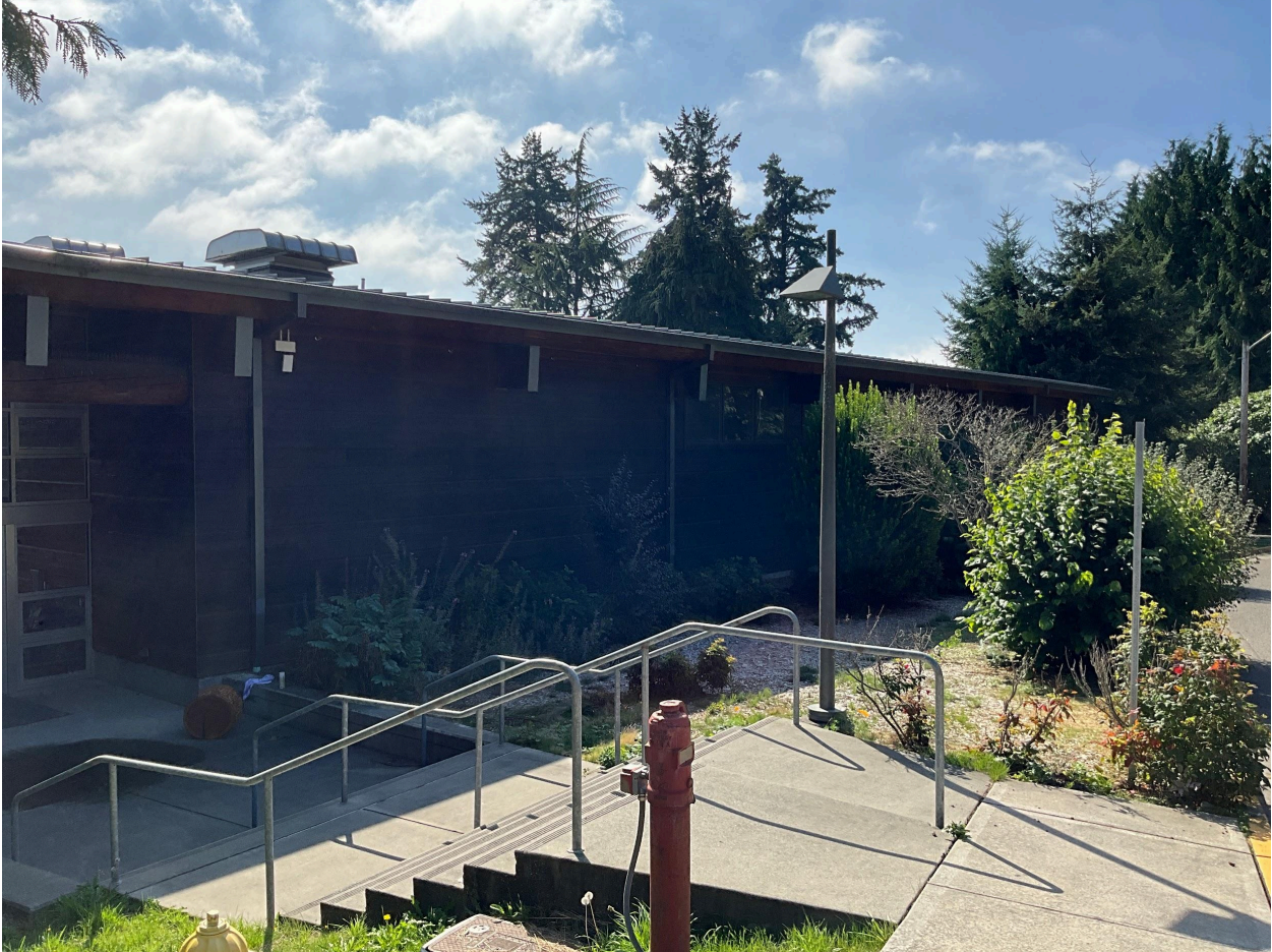
Solar/PV Installation Location - Ground-Level View of Roof #3:
