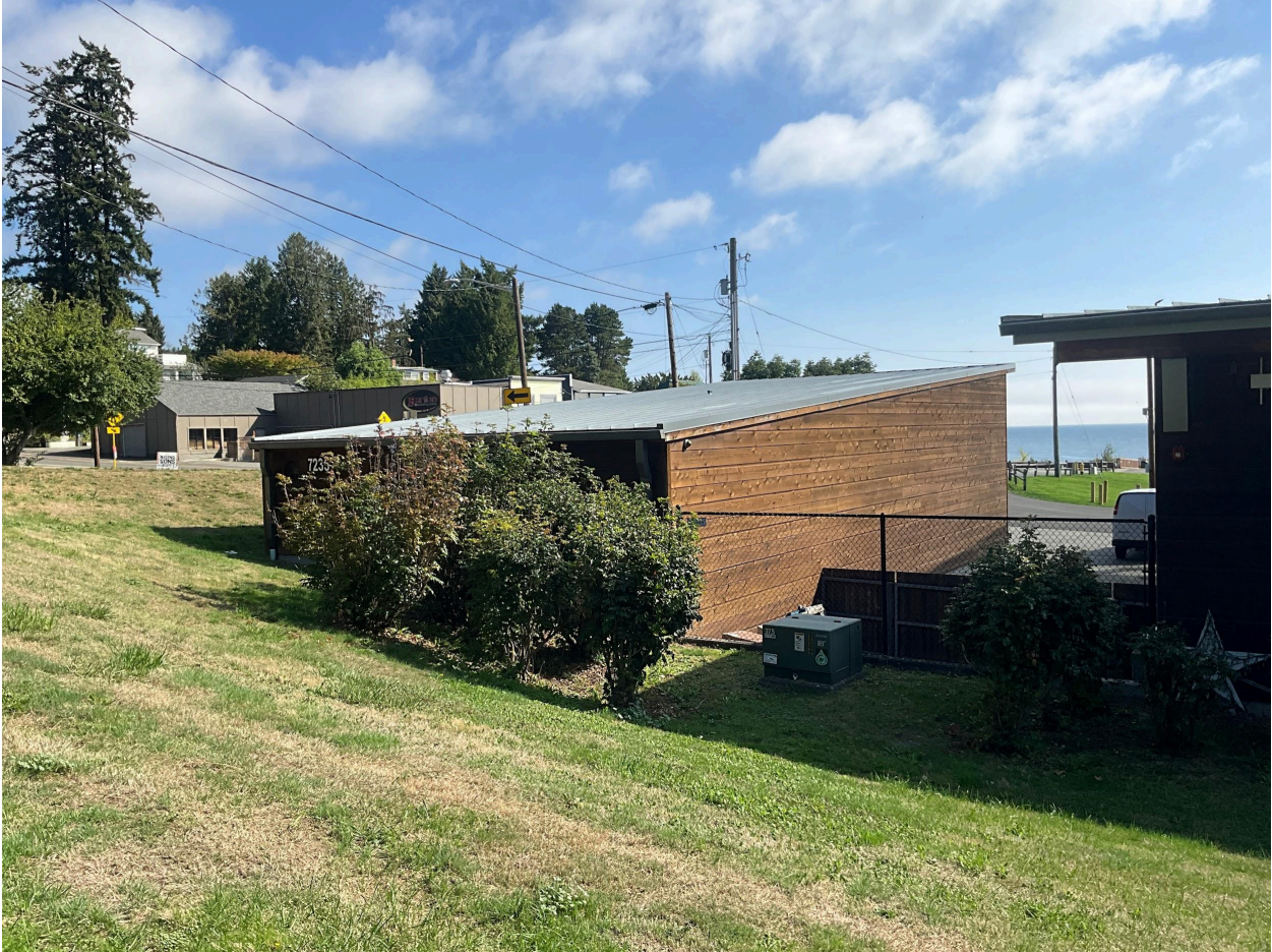
Solar/PV Installation Location - Ground-Level View of Roof #1:
