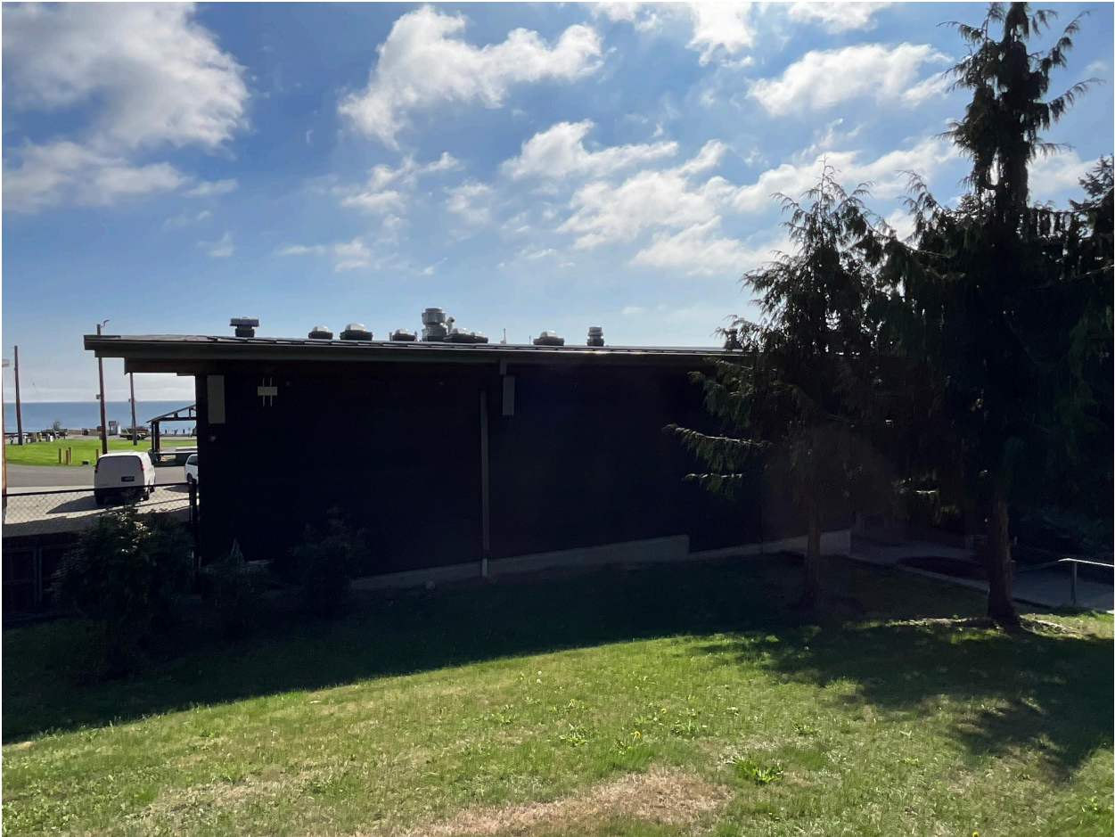
Solar/PV Installation Location - Ground-Level View of Roof #2:
